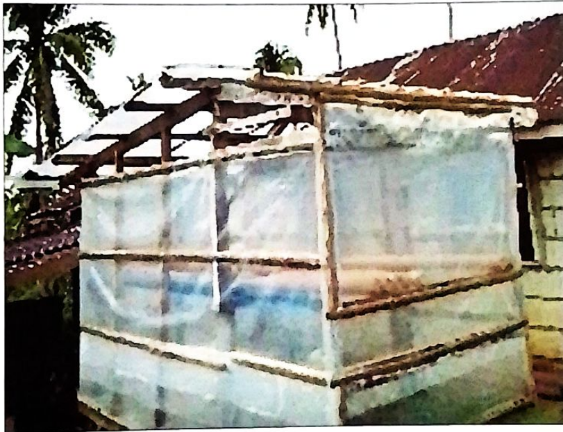
Figure 2. Greenhouse used as protective structure for the hydroponics system.
