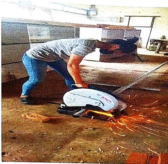
Cutting of GI pipe using cutoff saw
